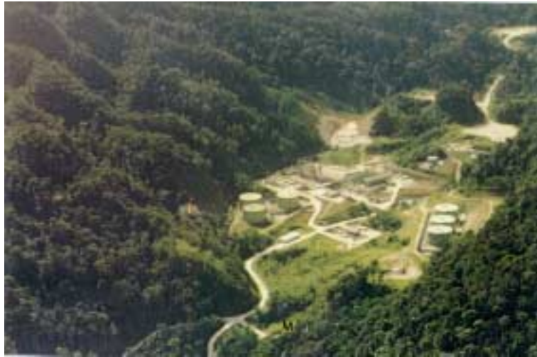
Figure 2 Kutubu Central Production Facility
